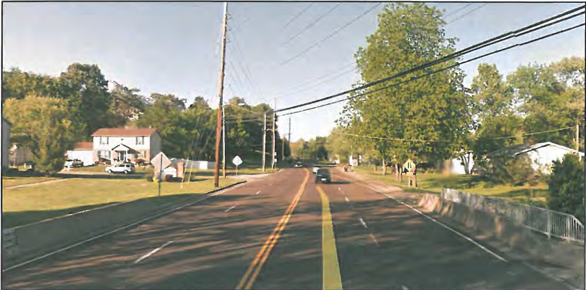
Figure 2: Old Lemay Ferry Road at Fawn Drive Looking North
